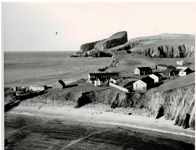
The ex-Naval huts at North Haven, home of the Bird Observatory between 1948 and 1969, with the mail-boat 'Good Shepherd' on the slipway and Sheep Rock (422ft) beyond.
