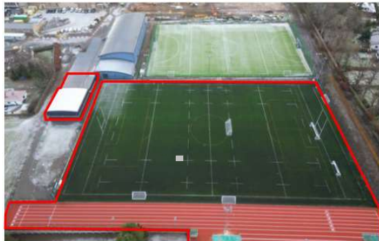
Sports Building Extension, 3G Pitch and Running Track
