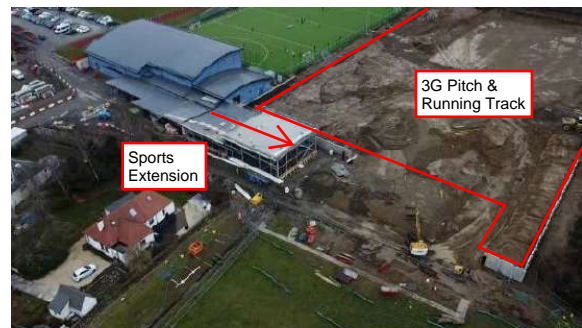
Earthworks commenced on the 3G pitch and running track
