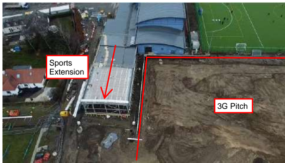
Sports Pavilion Extension and Retaining Wall Construction Underway.
