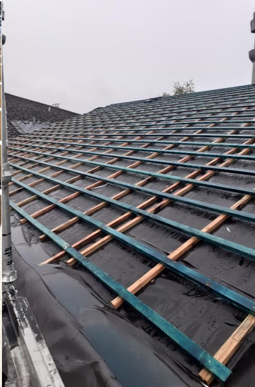
Roof Battens to take the roof tiles.
