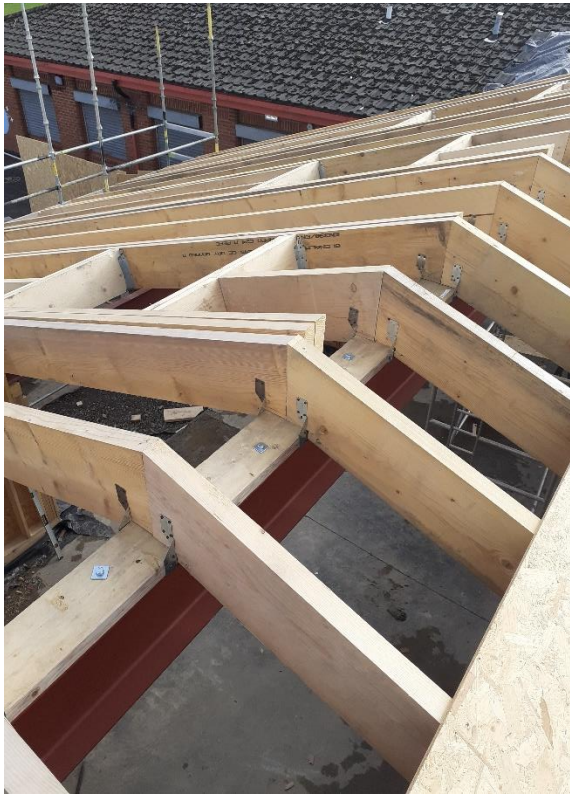
The Ridge (highest point of the roof)
