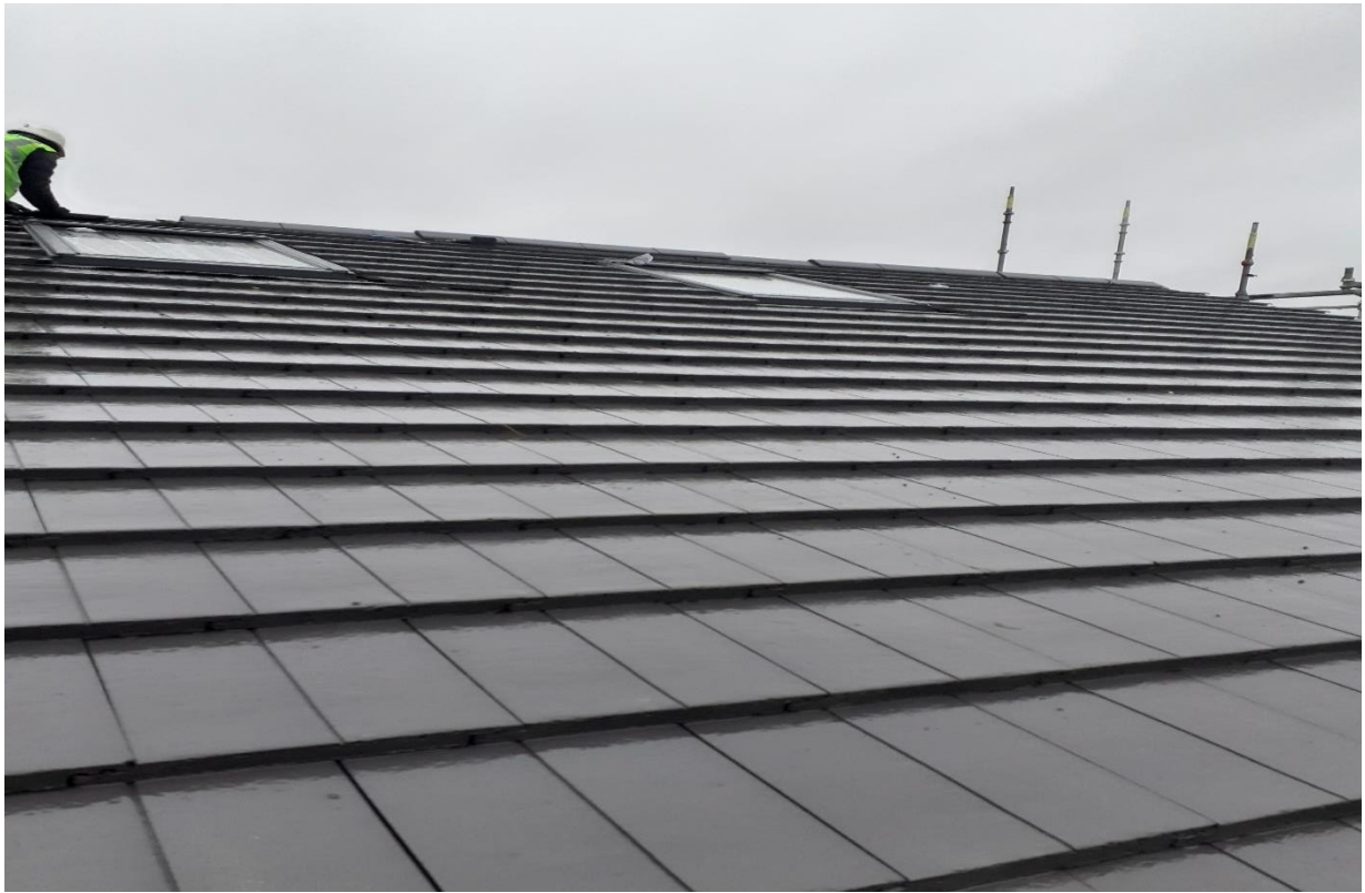
Roof Tiles and Roof Lights
