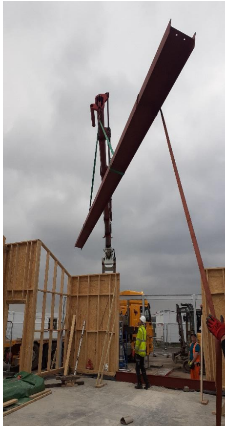
Steel at Roof Ridge
