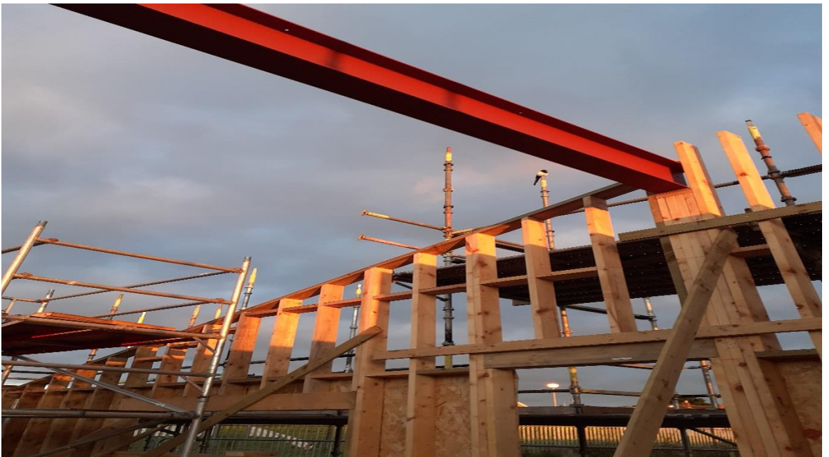
Steel for Roof Ridge
