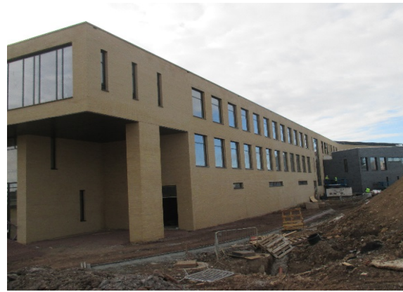
North West Corner
