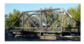
Truss bridges are one of the oldest types of modern bridges. The basic types of truss bridges shown have simple designs which could be easily produced by nineteenth and early twentieth century engineers. A truss bridge is economical to construct owing to its efficient use of materials.
