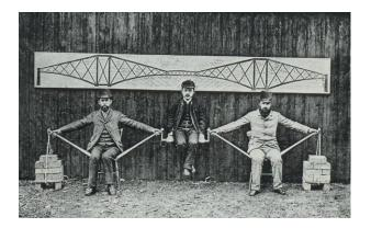
Benjamin Baker illustrated the structural principles of the suspended span cantilever in the photo on the left. The suspended span, where the man in the middle sits, is seen in the center. The need to resist compression of the lower chord is seen in the use of wooden poles while the tension of the upper chord is shown by the outstretched arms. The action of the outer foundations as anchors for the cantilever can be seen in the placement of the counterweights.
