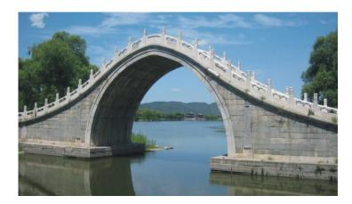
The arch pushes on to the ground at each end of the bridge. The arch can be made from either brick, stone, concrete, wood, iron or steel.
