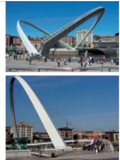
Millennium Bridge (2001), Gateshead, by architects Wilkinson Eyre and structural engineers Gifford The bridge pivots upwards to allow tall boats and ships to pass underneath
