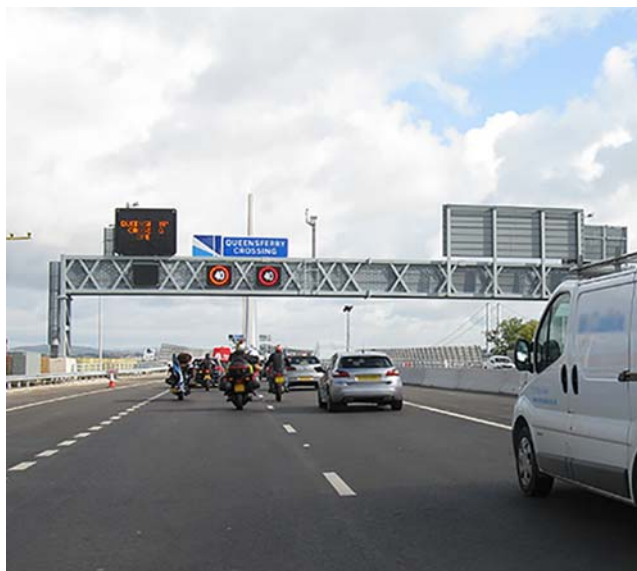
Variable speed limit, Queensferry Crossing. (Picture CC-BY-SA-2.0 M J Richardson/Geograph)
