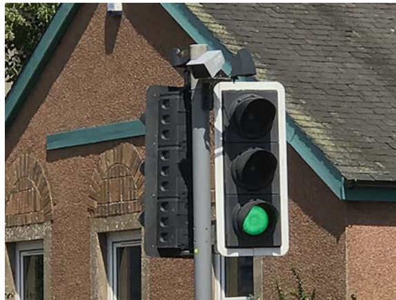
Photo of a 'smart' traffic light with pedestrian & traffic sensors
