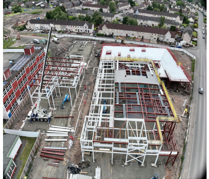
Aerial view of Orbiston site
