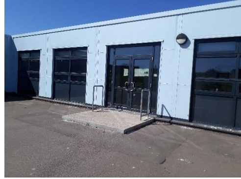
P1 Classroom Entrance
