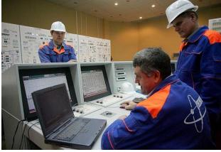
*Fig.* 10: *Russian contractors in the Bushehr nuclear power plant control room, setting up the SCADA systems.*
