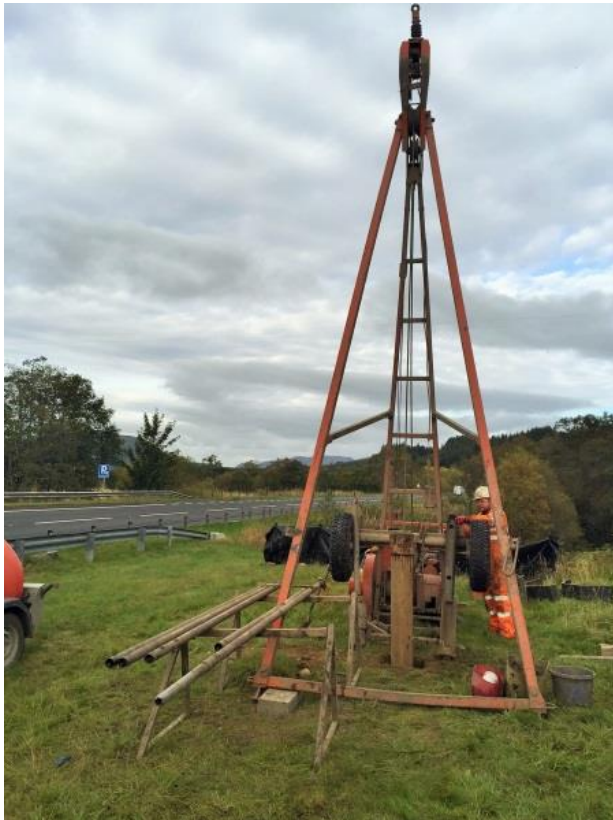
Light cable percussive rig
