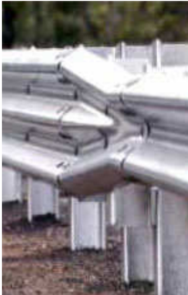
Galvanized steel crash barriers require no further finish for years of rust free service.
