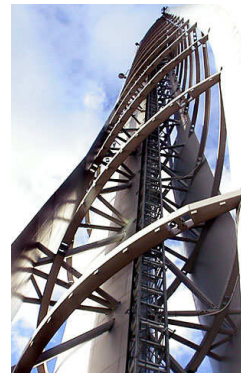
Detail of the steel structure in the Glasgow Science Centre Tower.
