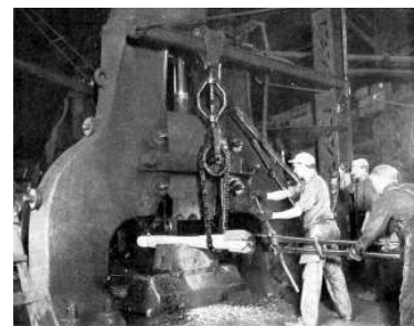
Drop forging used to form a steel axle for a railway carriage.
