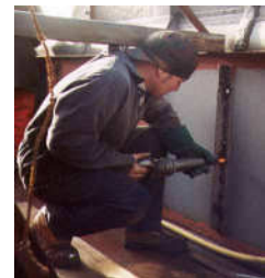
A hot steel rivet being formed by a pneumatic hammer.
