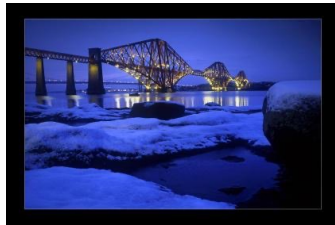
Forth Rail Bridge
