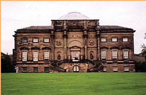
South front, Kedleston Hall, Derbyshire, designed by Robert Adam, c 1760 after the Arch of Constantine, Rome
