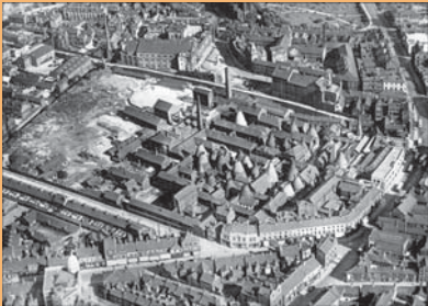
Aerial view of the Spode works, c1927, showing the bottle kilns
