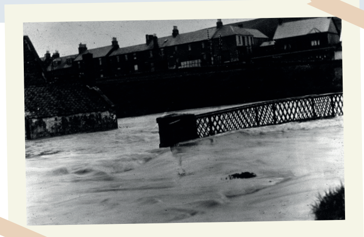
Flooding at Bonnybridge Ford, c.1893 Credit: unknown photographer via Falkirk Archives
