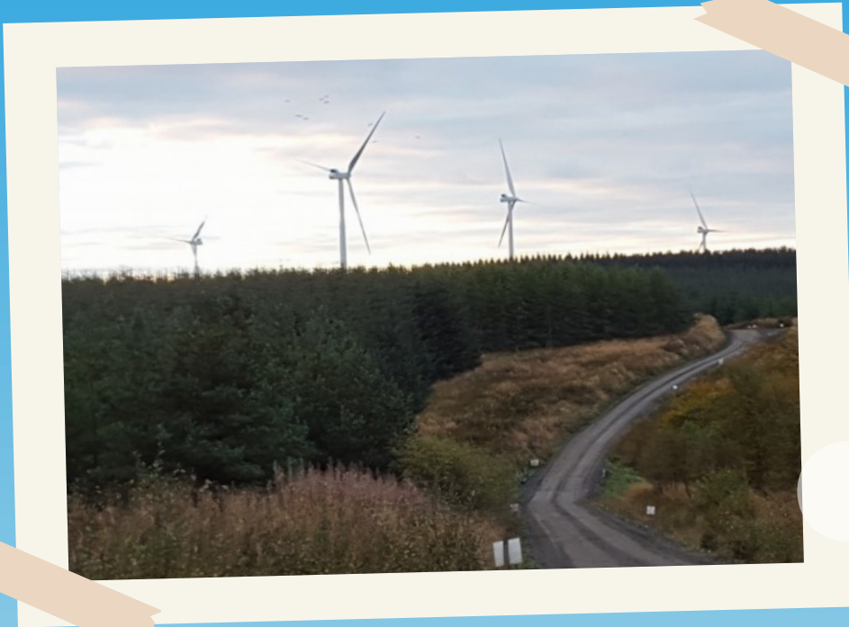
Burnhead Moss wind farm at Avonbridge. Credit: EDF Renewables
