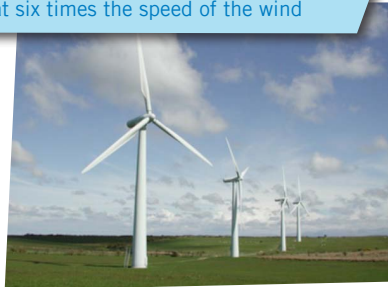
Wind farm turbines that have blades which turn at six times the speed of the wind
