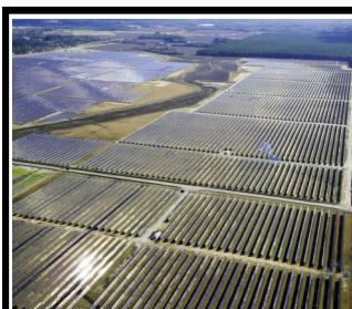
A solar farm
