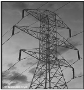
Resistance in electrical cables can prove costly.
