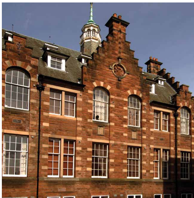
An old school now converted into flats
