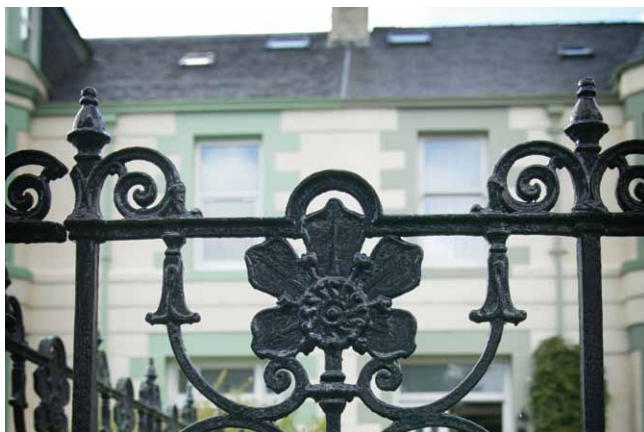
Finials and flower detail on cast-iron railings
