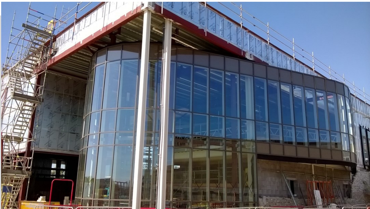
Progress - East Elevation - Sports Hall
